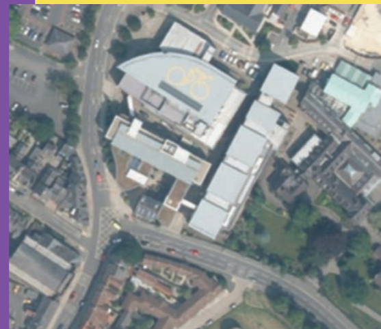
An aerial view of the Lord Mayor's Walk junction on the edge of the York St John campus
